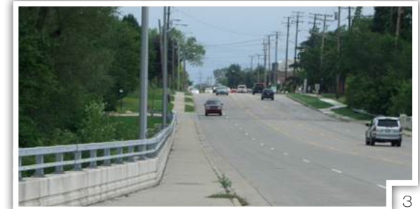
Bridge Over Rouge River
