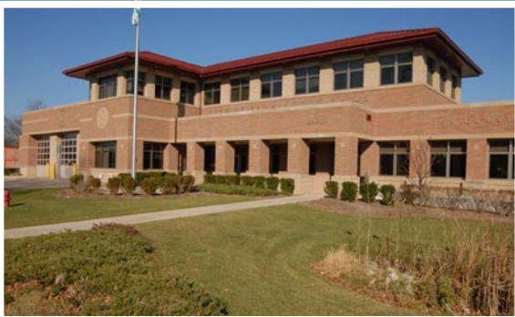
Fire Department / Community Center located along Grand River Avenue
