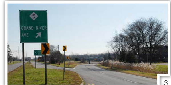
View driving south before interchange
