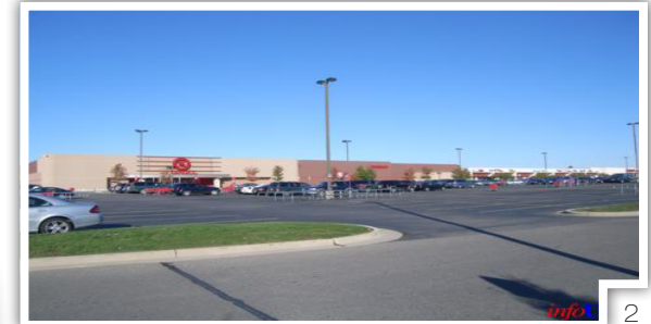
View facing Target development
