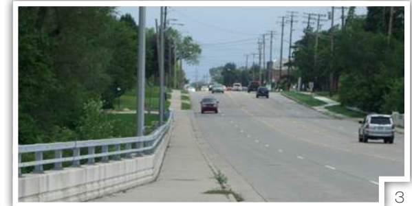
Bridge Over Rouge River
