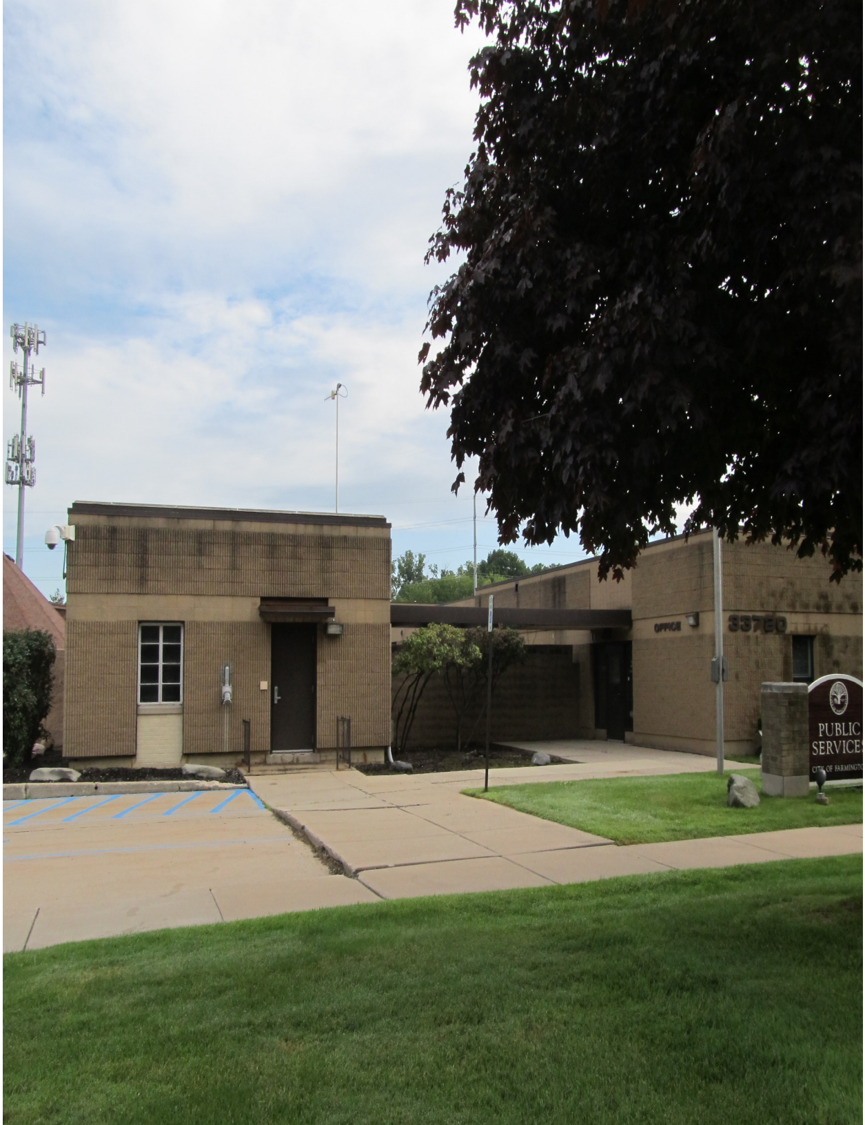
Farmington Pump Station located at 33720 West 9 Mile Road, Farmington Michigan.
