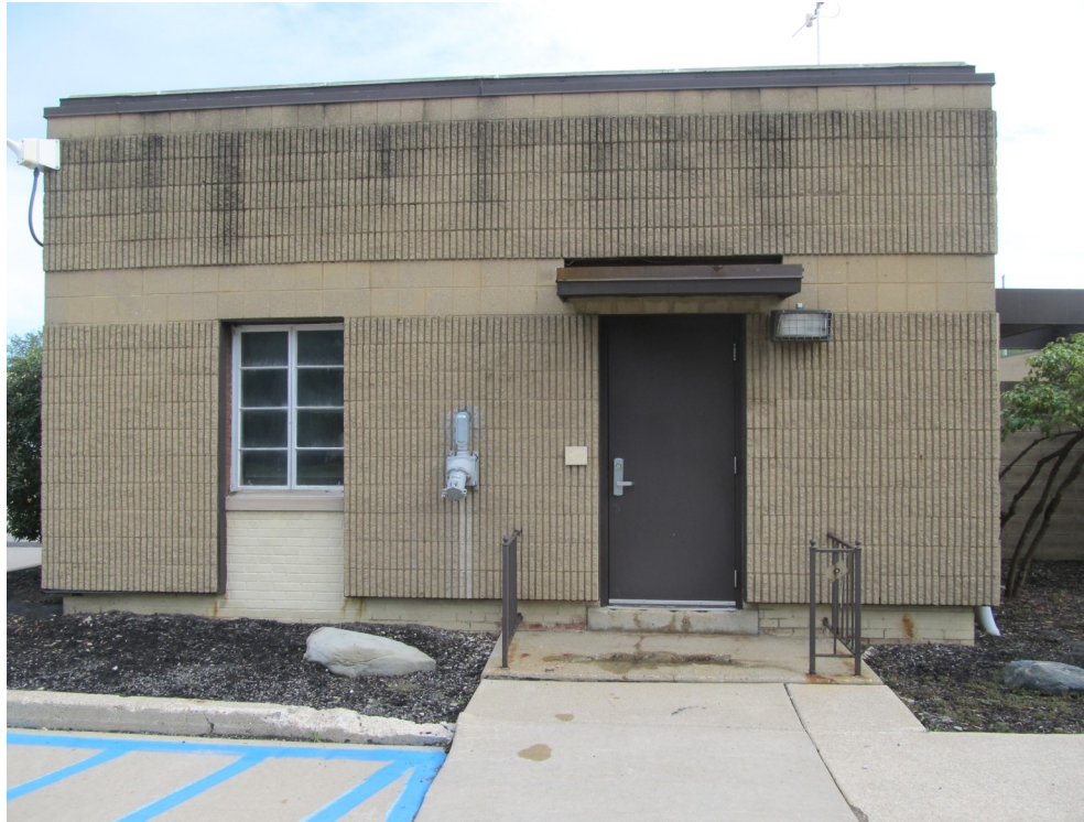
1) The station houses pumps, controls, and piping.
