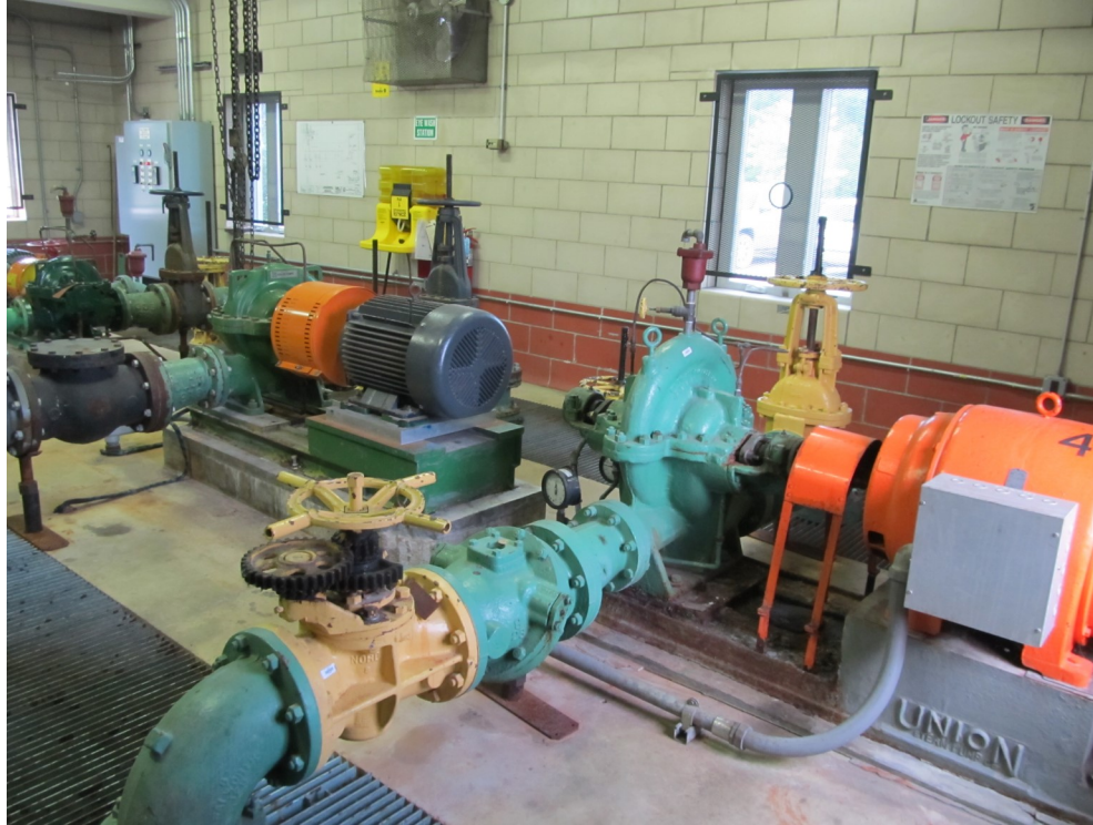
8) There were no leaks observed during the inspection.
