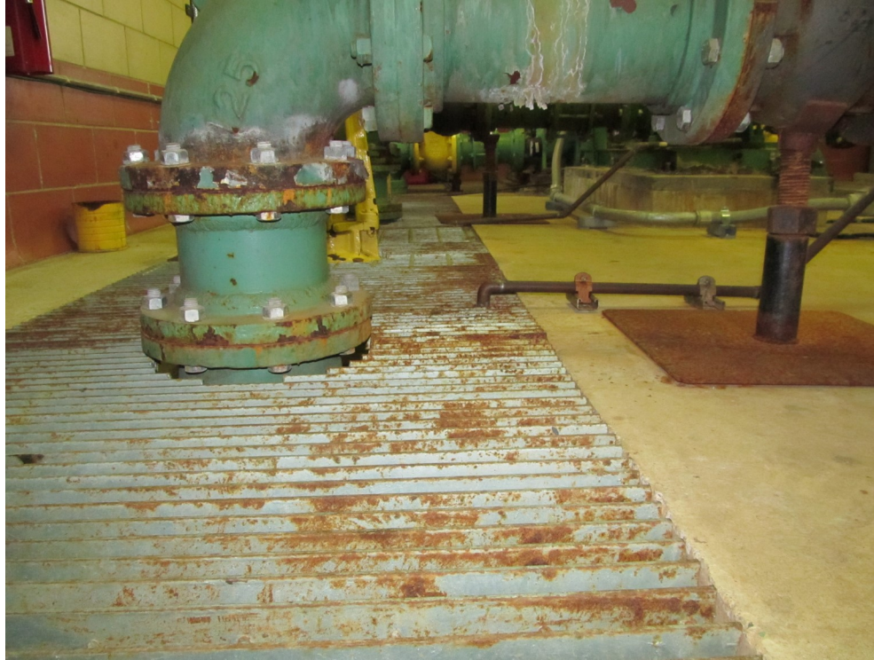
20 Grating under influent piping.
