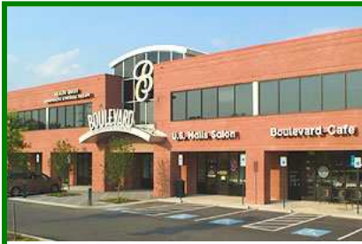
Example of office building with ground floor service uses
