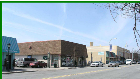
Example of inappropriate building line – inconsistent building line
