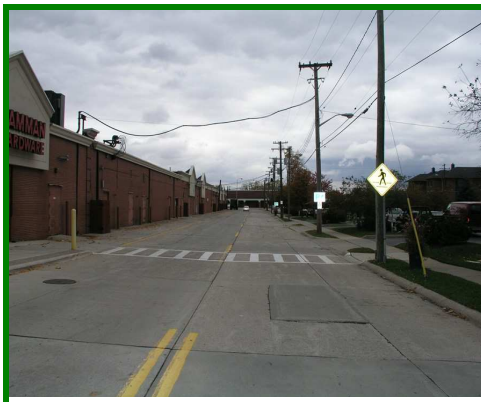
Existing Orchard Street designed as a service alley.
