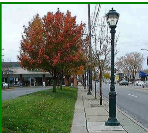
Existing ornamental street lights in downtown Farmington
