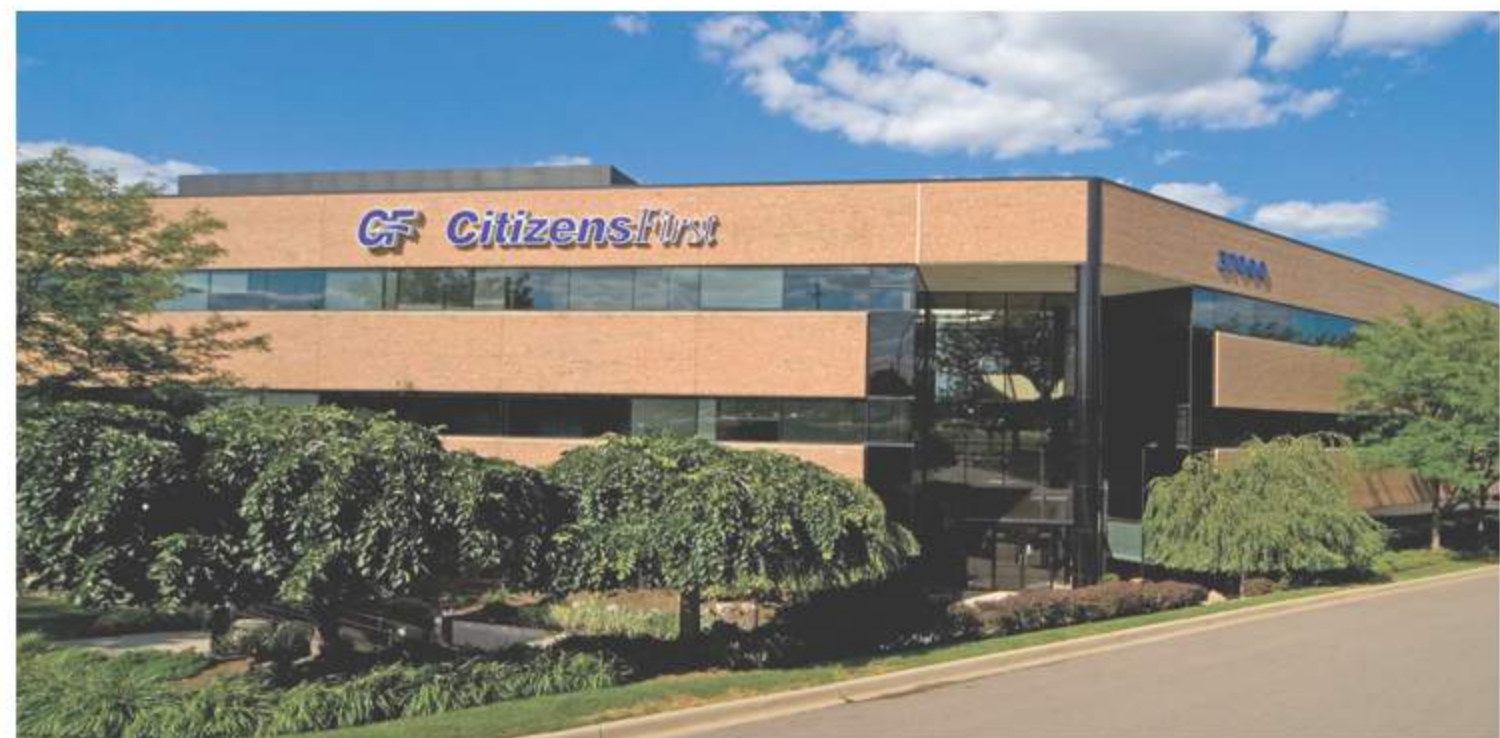
EXISTING OFFICE BUILDING ACROSS GRAND RIVER AVENUE
