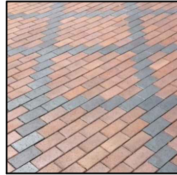
RUNNING BOND BRICK PAVERS WITH 'ARGYLE' STRIPING (SE CORNER OF GRAND RIVER AVE. AND LIBERTY ST.)
