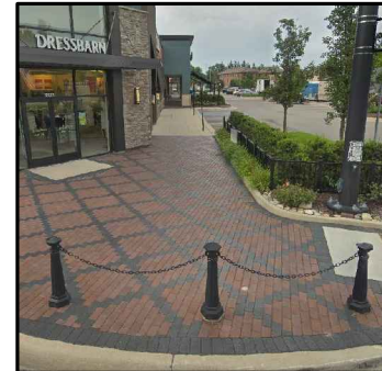
BOLLARD: FAIRWEATHER SF, MODEL CU-CB-B CAST DUCTILE IRON BOLLARD WITH NON-STANDARD BREAKAWAY IMPACT MOUNTING CHAIN: CREATIVE PIPE
