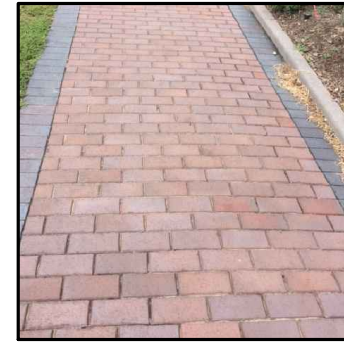
RUNNING BOND BRICK PAVERS (OAKLAND ST. & FARMINGTON ST. PLAZAS ON WEST SIDE OF INTERSECTION)
