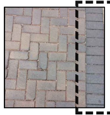
SOLDIER COURSE ADJACENT TO HERRINGBONE BRICK PAVER CROSSWALK (OAKLAND ST. & FARMINGTON ST. CROSSWALK, ON WEST SIDE)
